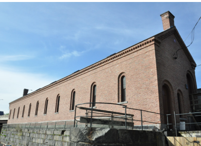
The Pawtucket Gatehouse can raise and lower the dam to control how much water enters the city's industrial canal system.
