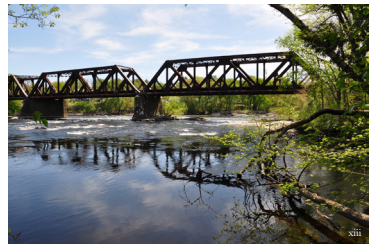
A railroad bridge crosses the river in Bedford, NH.
