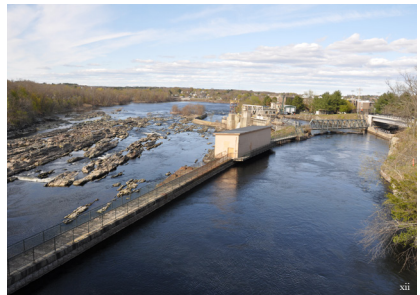
The Northern canal (foreground) diverts water from above the dam to create a more navigable and useable channel than the rocky riverbed below.
