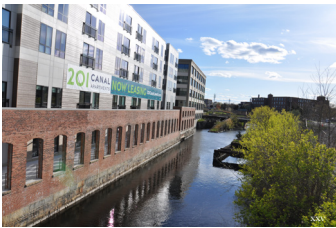
Many old mill buildings in Lowell have been put to adaptive reuse such as condominiums.
